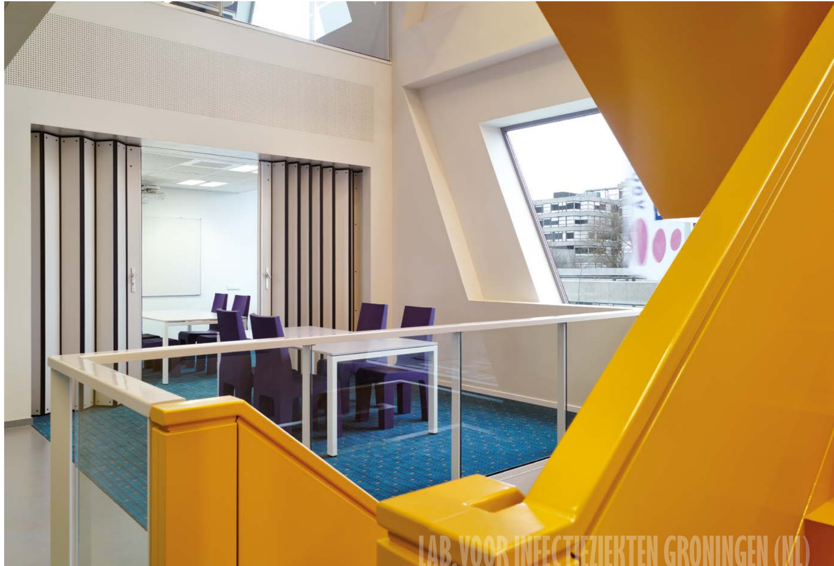
6 a Duplo wall with centre closure, sufficient privacy thanks to the sound insulation rating of \pm 43 dB.
